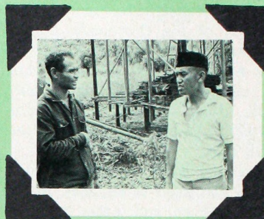
Nias and Isack at the Loksado building project
